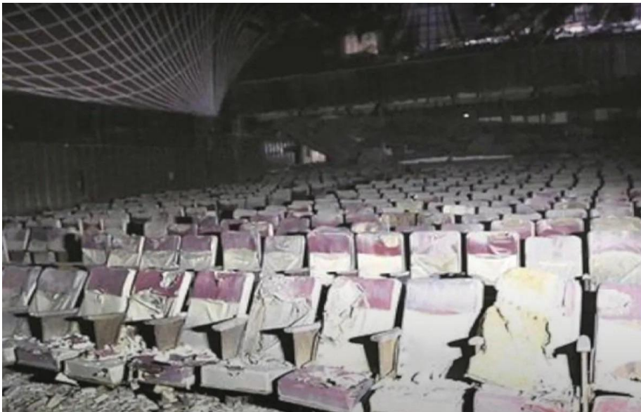
Picture 1: The charred seats of Uphaar (Source: HT)
